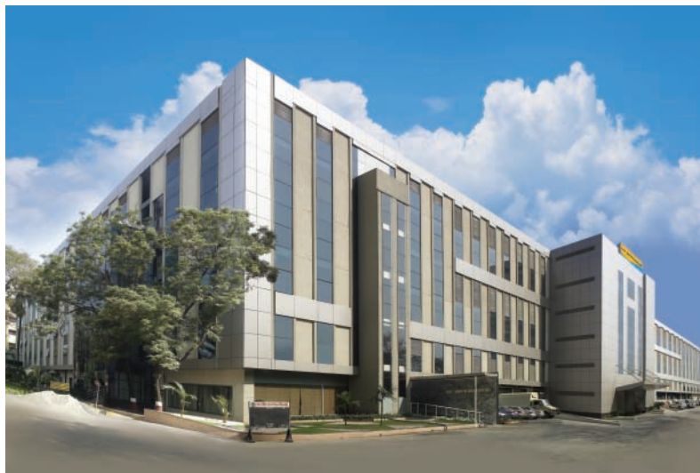
Switchgear Factory, Mumbai
