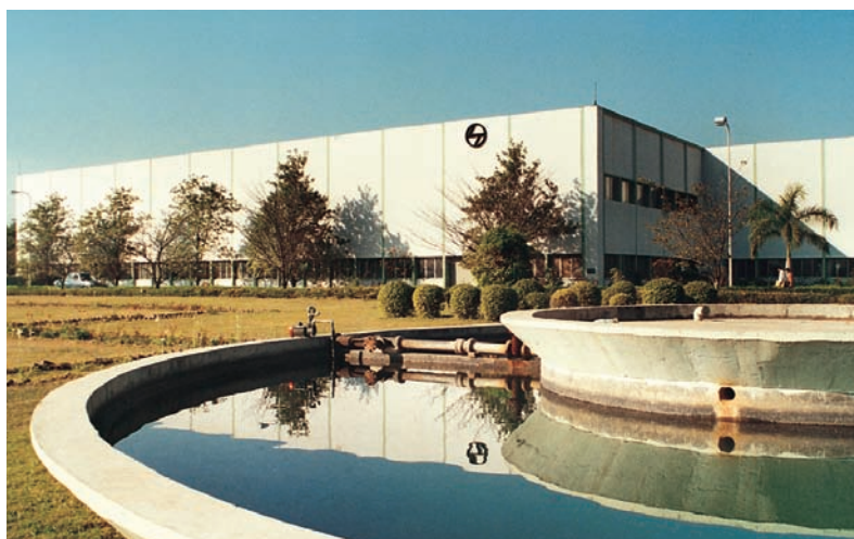
Switchgear Factory, Ahmednagar
