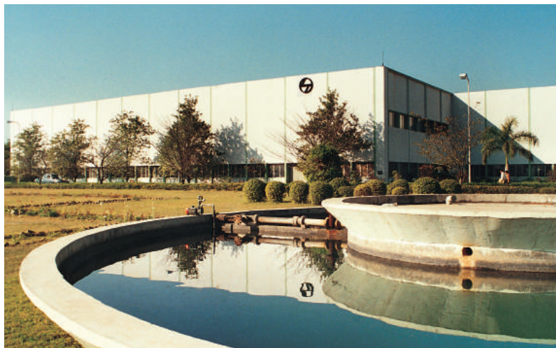
Switchgear Factory, Ahmednagar
