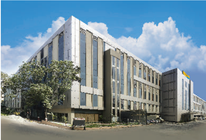
Switchgear Factory, Mumbai
