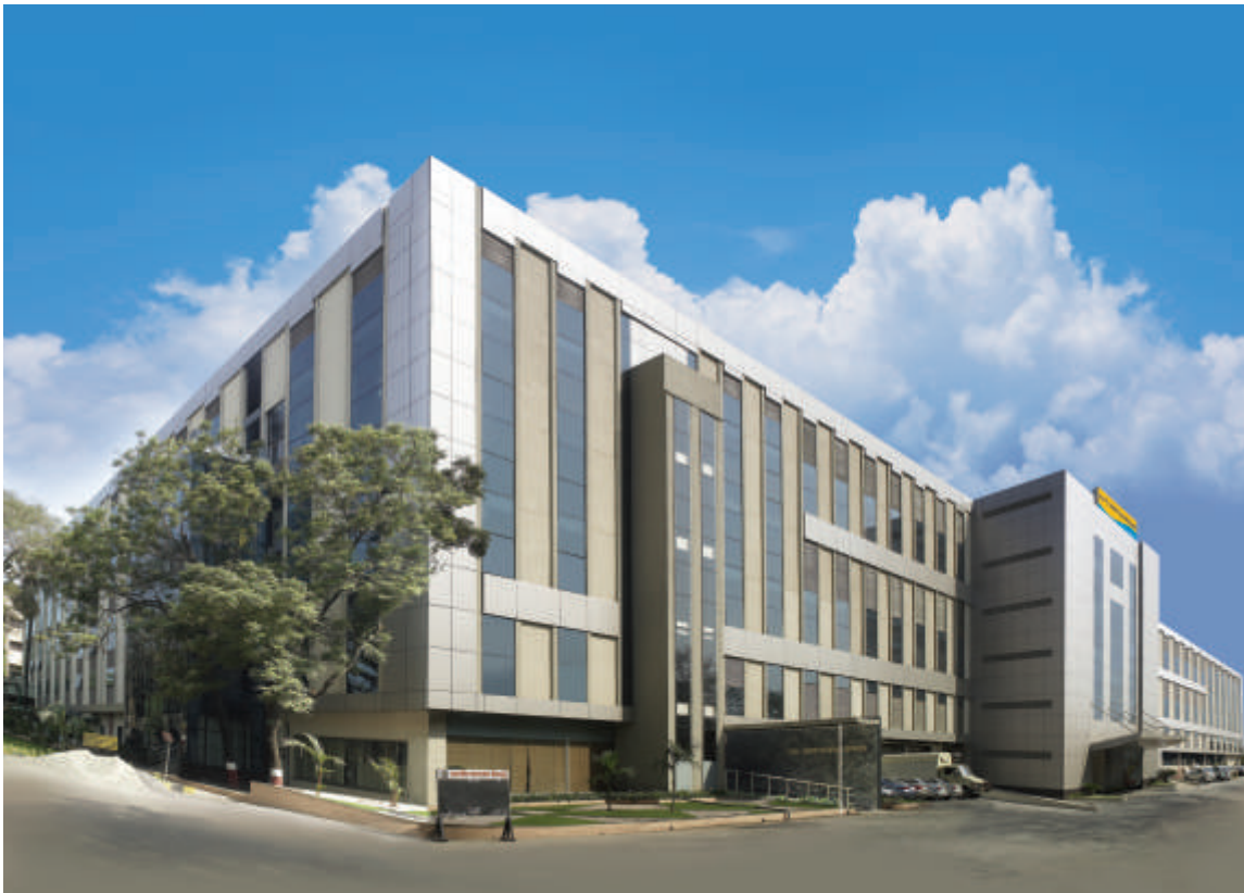
Switchgear Factory, Mumbai
