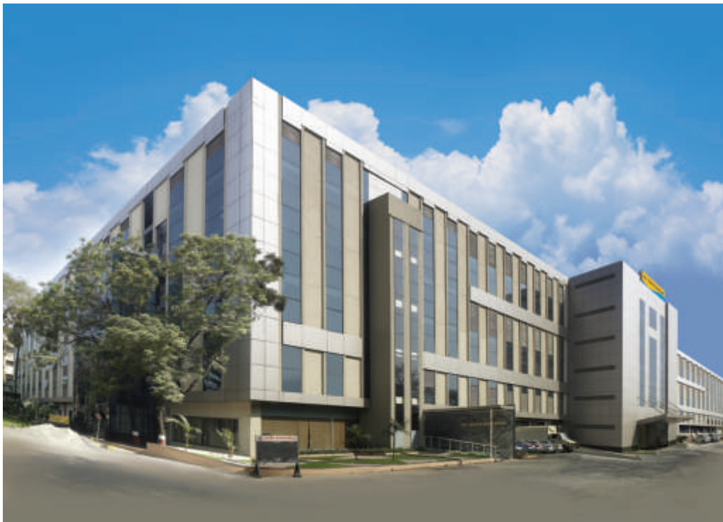
Switchgear Factory, Mumbai
