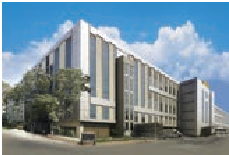
Switchgear Factory, Mumbai
