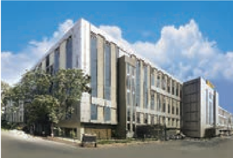
Switchgear Factory, Mumbai
