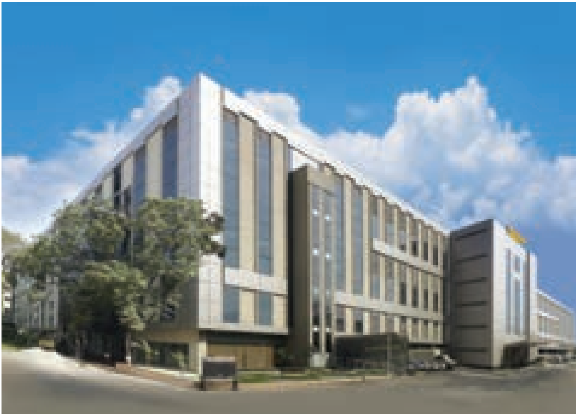
Switchgear Factory, Mumbai
