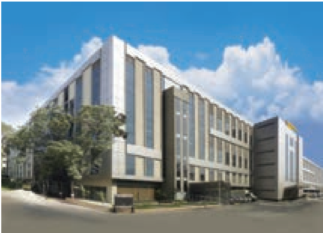
Switchgear Factory, Mumbai
