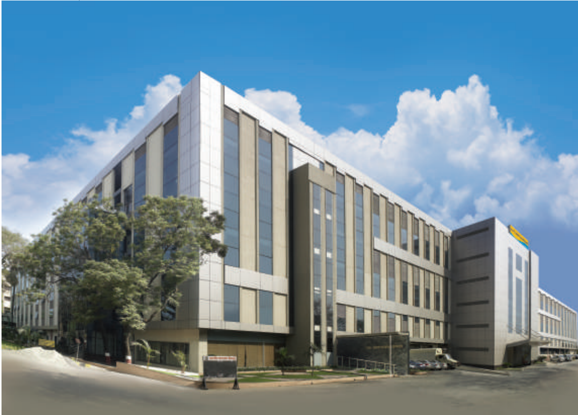
Switchgear Factory, Mumbai
