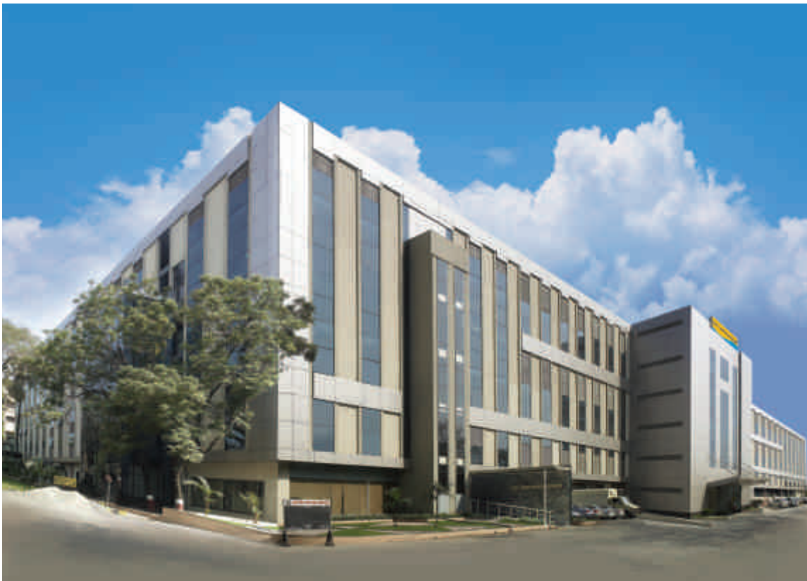
Switchgear Factory, Mumbai
