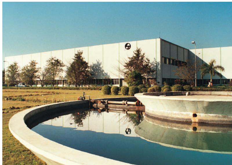
Switchgear Factory, Ahmednagar
