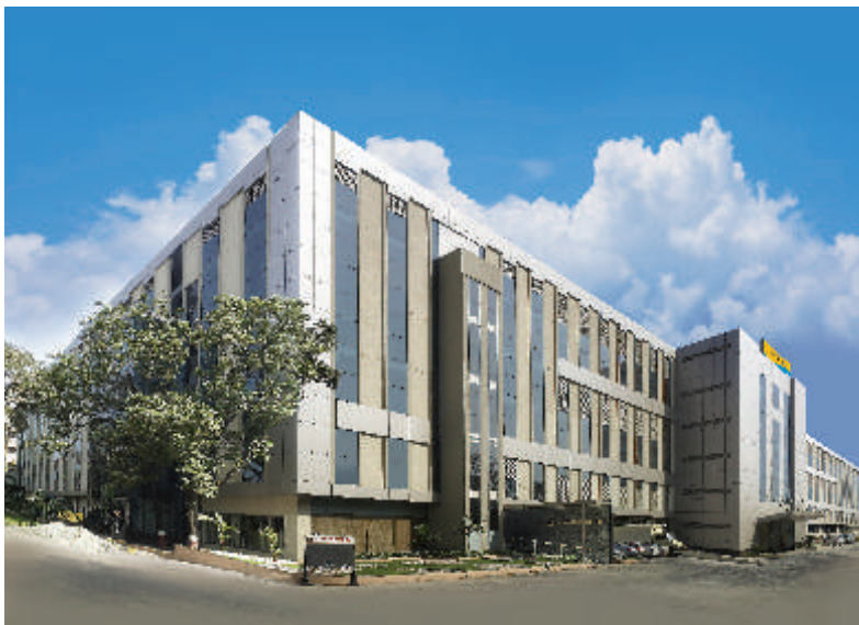
Switchgear Factory, Mumbai
