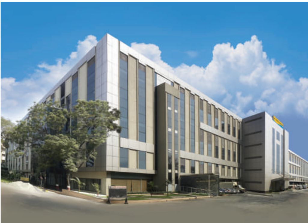
Switchgear Factory, Mumbai
